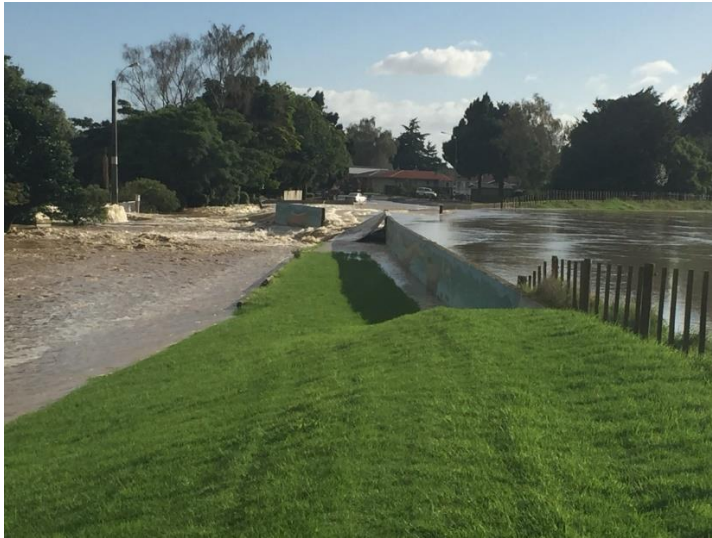
Figure 20: The breached Floodwall at Edgcombe, looking downstream; image file date-stamped 08:35 6 April, some 5 minutes after the breach (Source: Bay of Plenty Regional Council Contractor, 2017)
