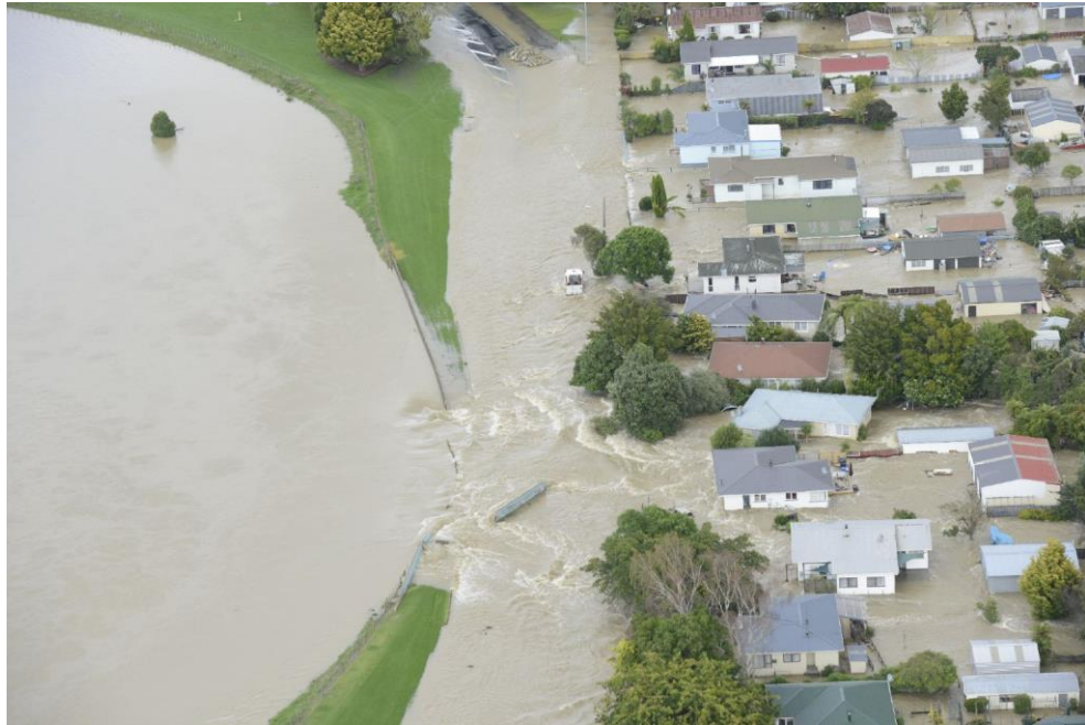
Figure 21: The breached Floodwall at Edgecumbe, at 11:00 6 April. Some of the wall sections can be seen still standing upright in the floodwaters some 2.5 hours after the initial breach (Source: Bay of Plenty Regional Council, 2017)
