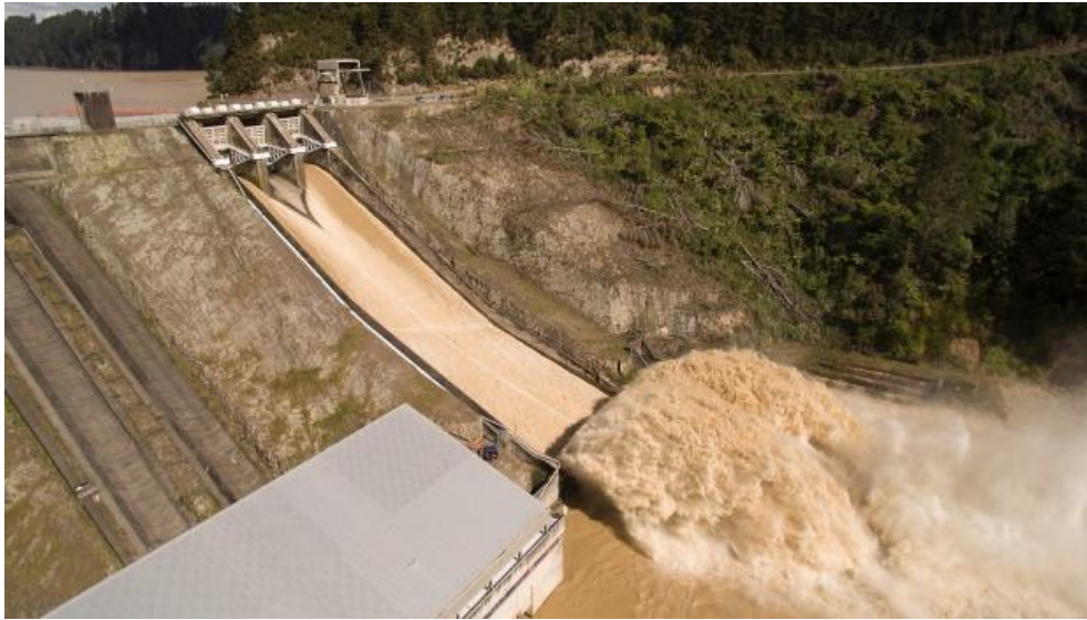
Figure 25: Matahina Dam spillway operating during April 2017 flood (Source: Chris McKeen/Fairfax NZ)
