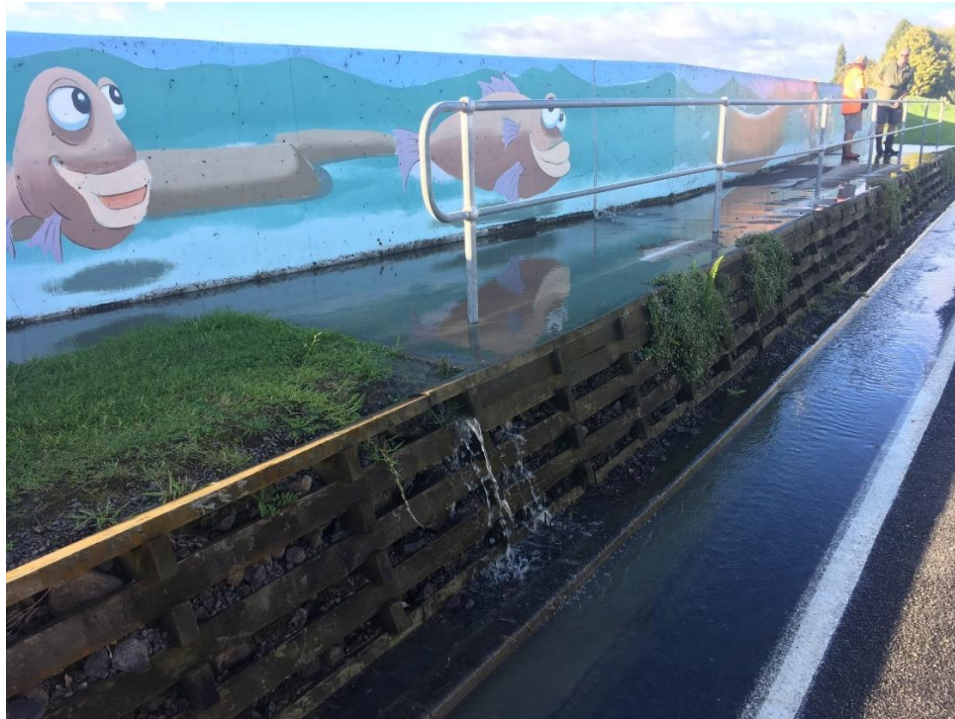
Figure 18: The Edgecumbe Floodwall, known locally as ‘The Painted Wall’, at 08.14 on 6 April, 15-20minutes before the breach (Source: Bay of Plenty Regional Council, 2017)
